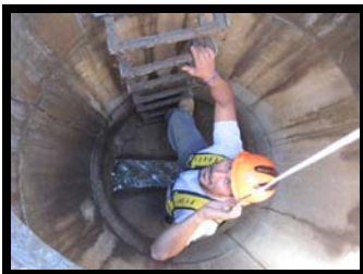
New Employee, Dave Magliocco practices being lowered into a manhole.
